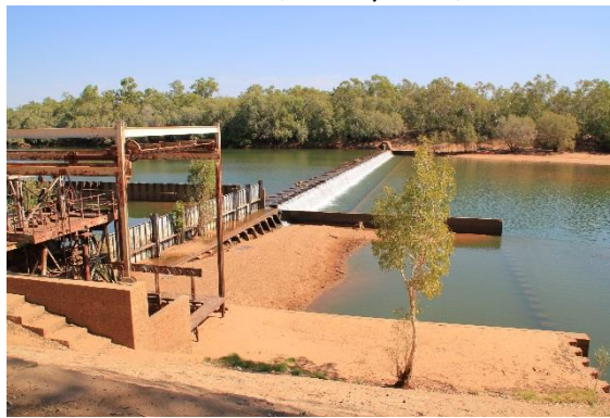
Camballin Weir, Fitzroy River, WA
