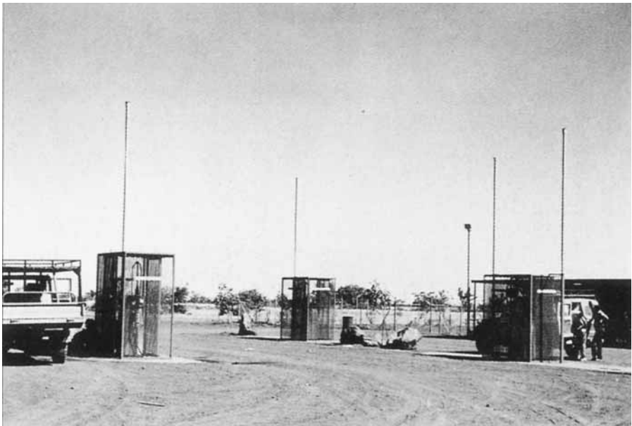
Plate 1: Caged bowsers at a roadhouse in Western Australia
