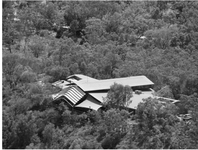
An aerial view of the Nitmiluk Visitor's Centre designed in the shape of Nitmi cicada. Photo Ray Whear.
