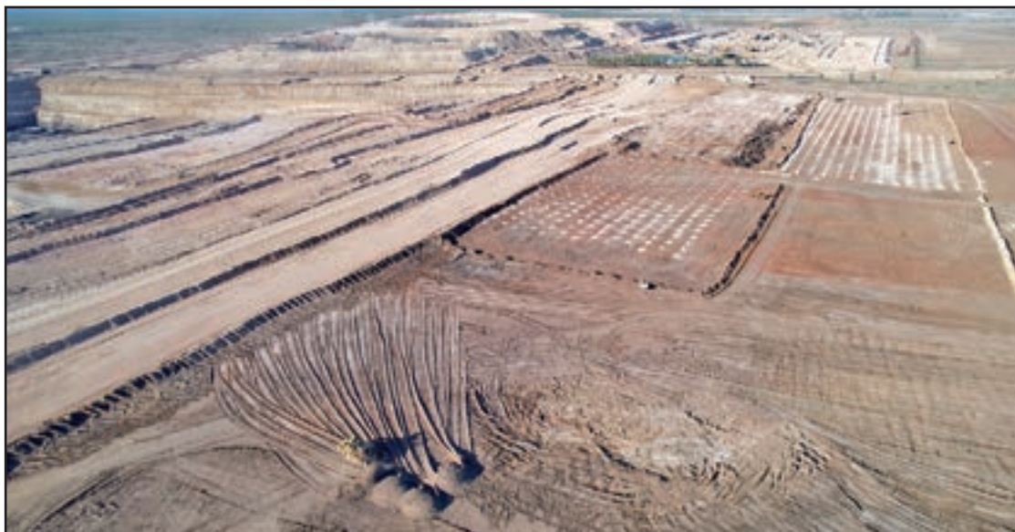
Bravus (formerly Adani Australia) is pushing on with construction of the Carmichael coal mine in Central Queensland despite opposition from traditional owners.
