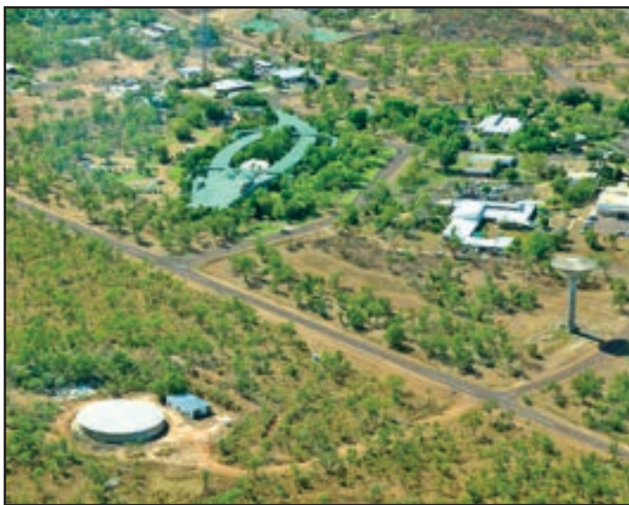
An aerial view of Jabiru township.
