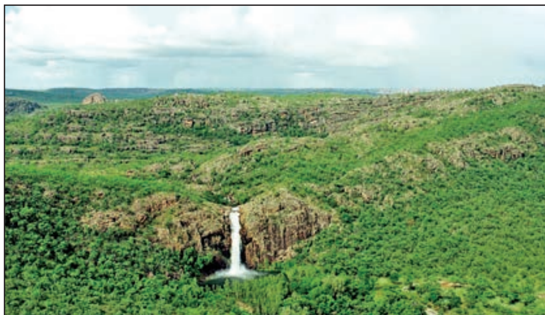
Parks Australia is facing court action following the construction of a walking track in Kakadu at Gunlom that was built without permission or certification from the Indigenous custodians.
