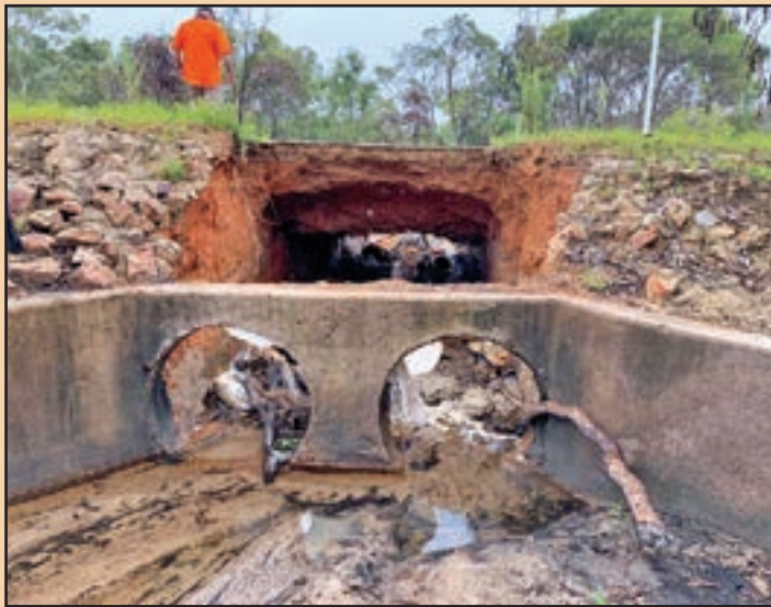
Lockhart River road is under construction, but the COVID-19 pandemic will probably mean delays.
