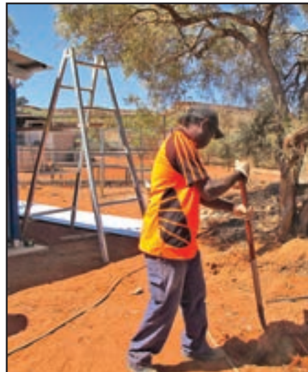
Training and employment of local Aboriginal people are key components of the building program.
