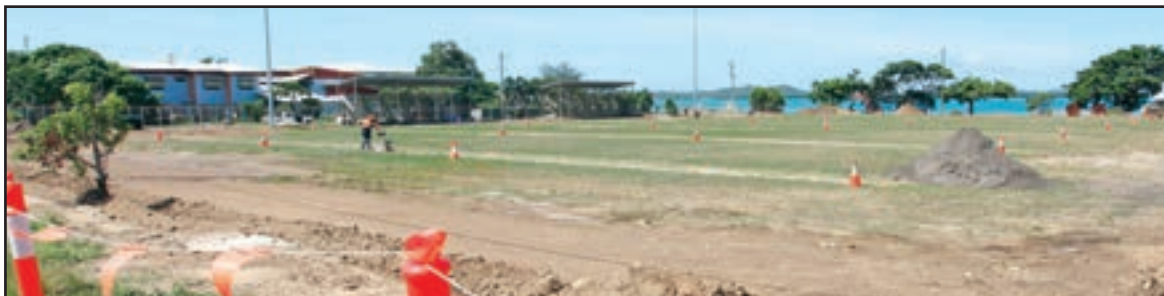
Ken Brown Oval on Thursday Island during May, in the middle of upgrades.
