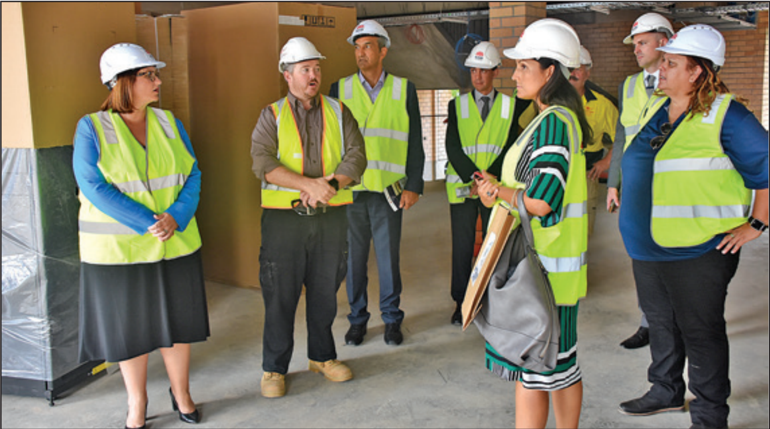
Mark West, project manager with PSG Holdings, gives a tour of the work being done at the Kimberwalli Centre.
