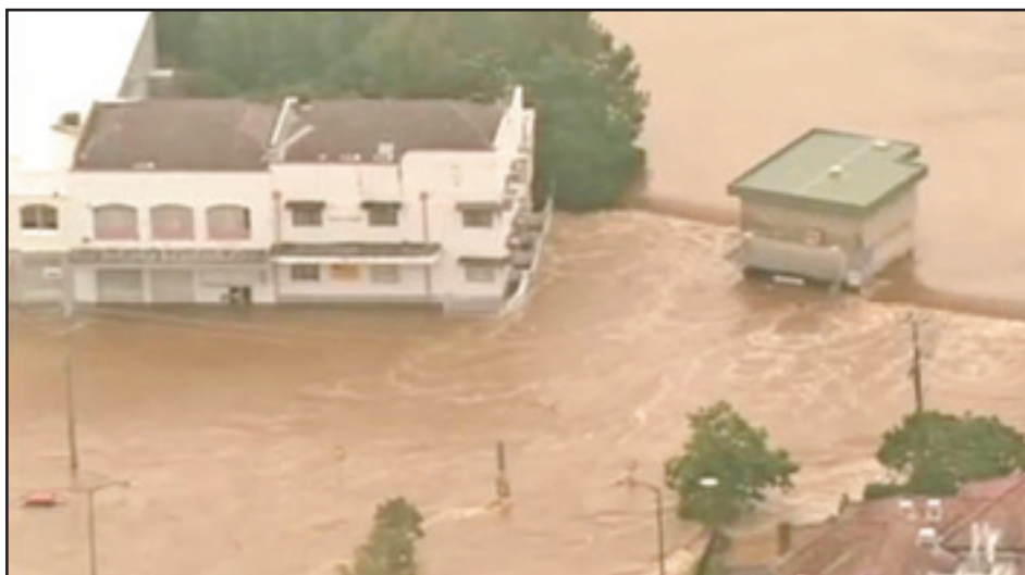
We at the Koori Mail know first-hand how bad the flooding was. Pictured is our head office in Lismore, with flood waters pouring over the adjoining levee wall. Staff worked long hours in difficult circumstances to put out this edition.
