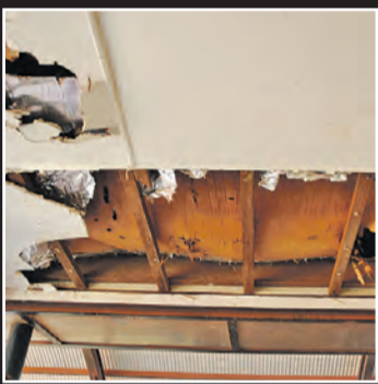
Damage to the eaves of the West Arnhem Shire office in Maningrida has exposed asbestos.
