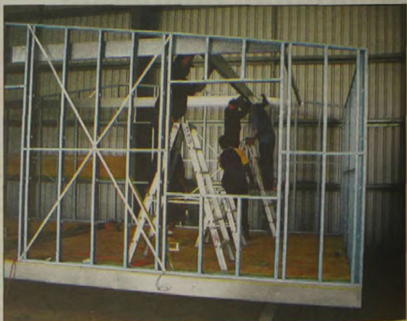
Batchelor students assembling a steel-framed structure.
