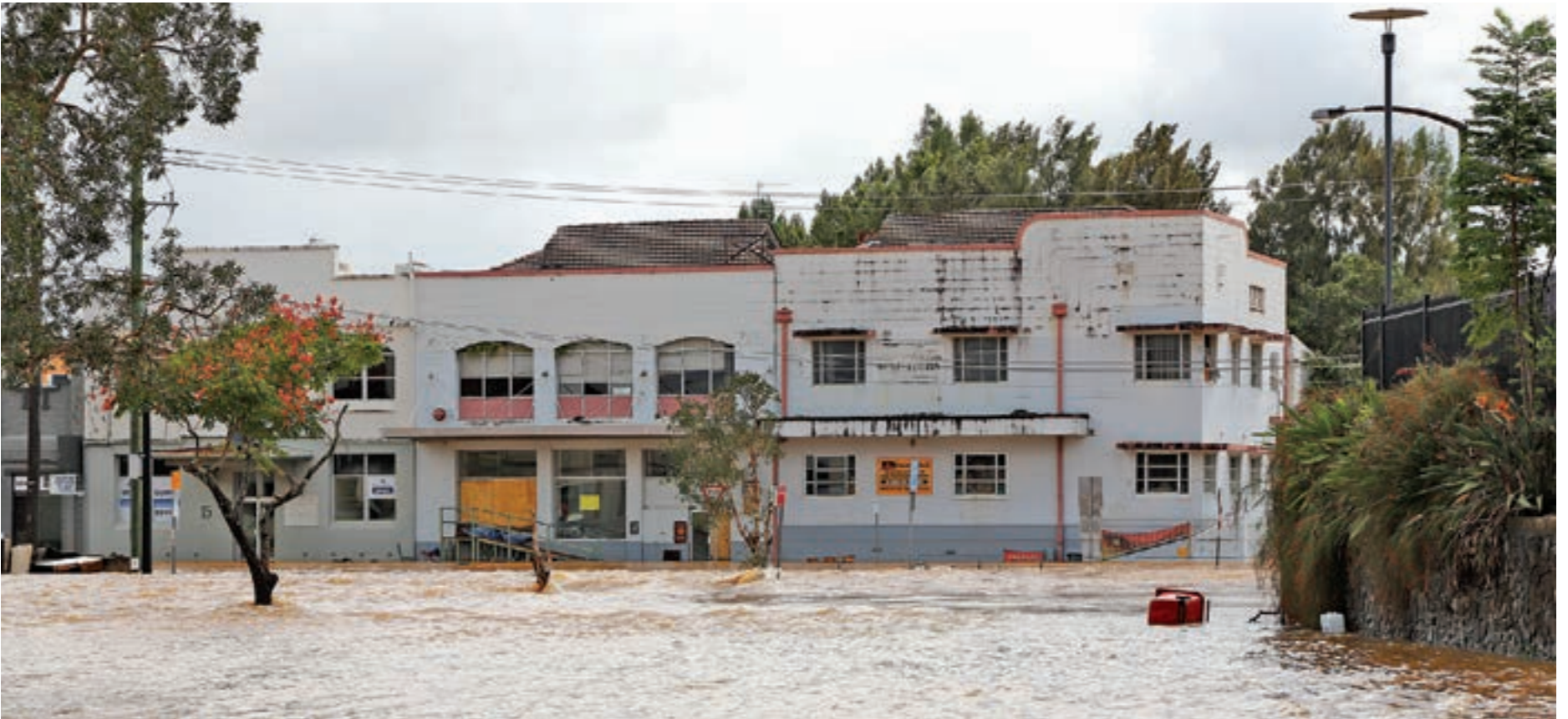
Here we go again! The Koori Mail building begins to flood for the second time on March 30. Pictures: Nick Paton
