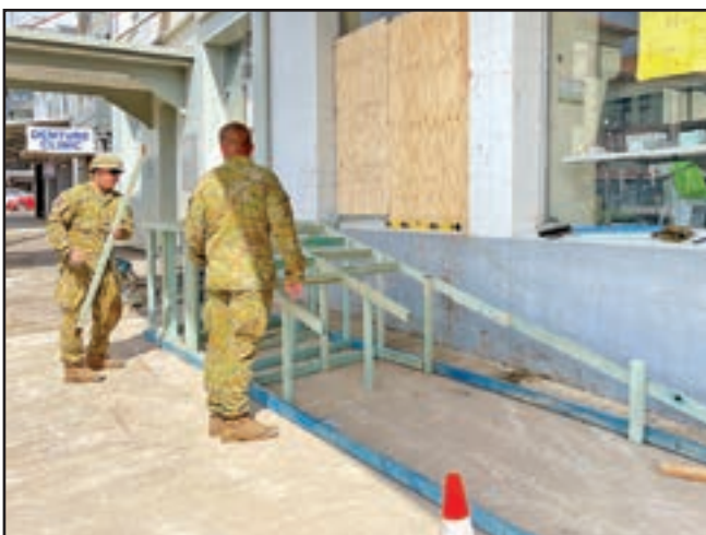
The ADF assisted with building a ramp for access to medical supplies and a treatment area.
