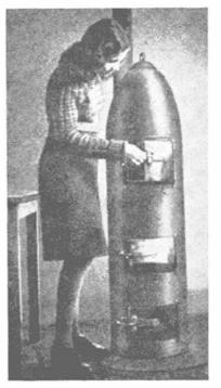
Even unexploded bombs are being used in Germany commercial products because of the shortage of materials. A Hamburg firm is removing the explosive 1000-pound from dud bombs and rebuilding the shells into stoves. Hinged doors permit fuel to be added and ashes to be taken out.
