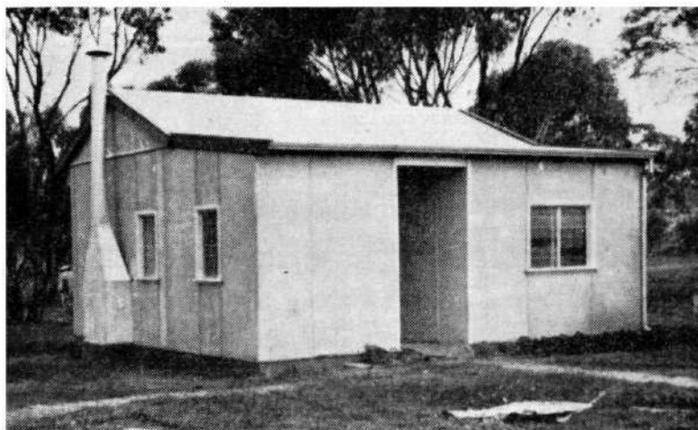
View of 2 cottages built by Mr. T. Cowcher, Geeralying for native employees
