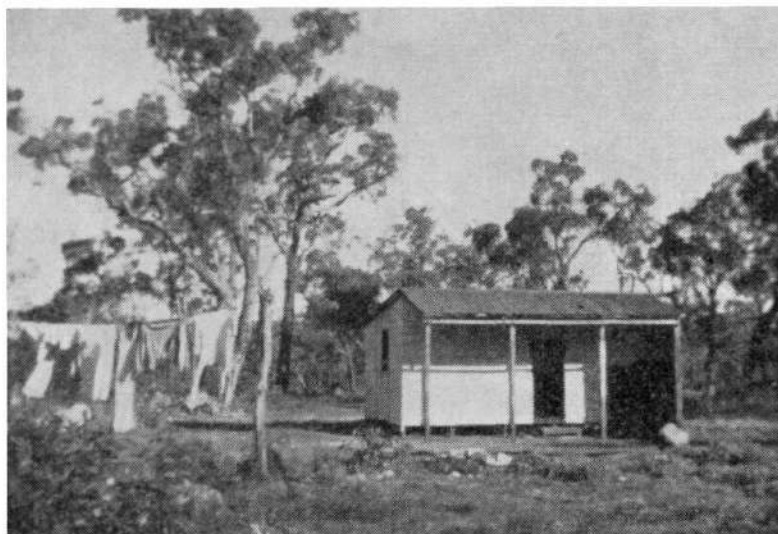
Cottage renovated, repaired and painted by Mobile Welfare Officer
