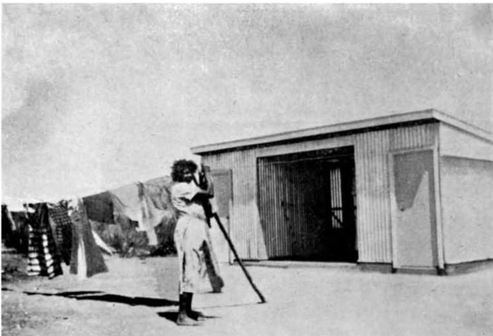
The ablution-laundry block with shower room each end and copper and troughs in central section
