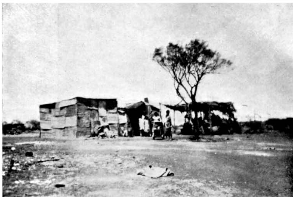
A native camp before re-erection
