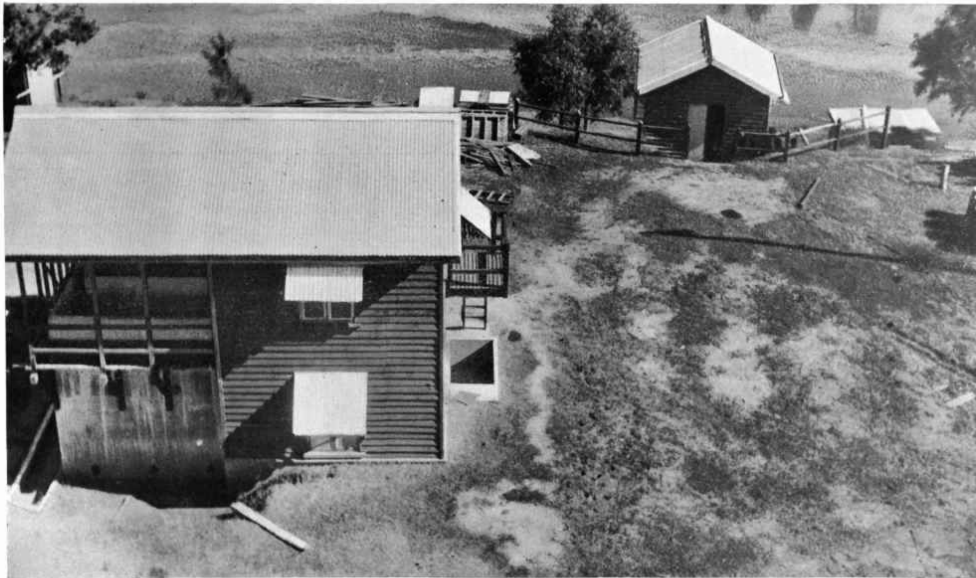
Treatment Plant, Woorabinda Water Supply.
