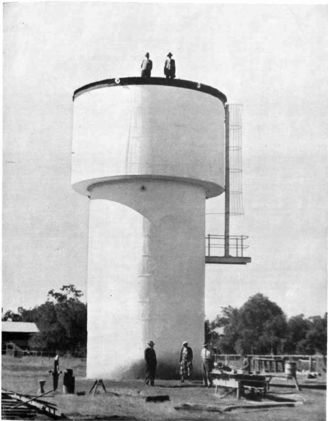
Concrete Water Tower, Woorabinda Water Supply.
