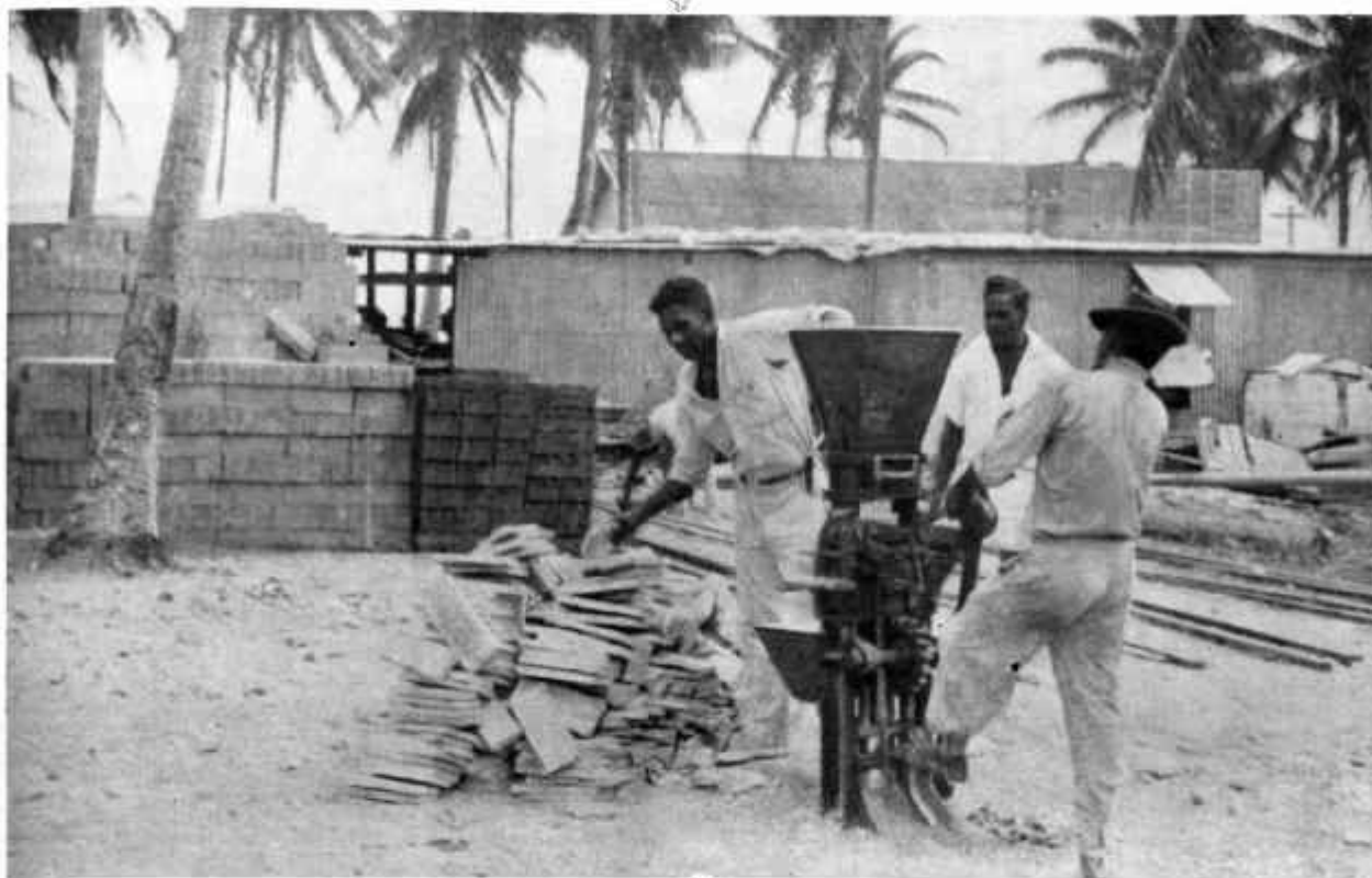
Concrete Brick Manufacture, Palm Island Settlement.
