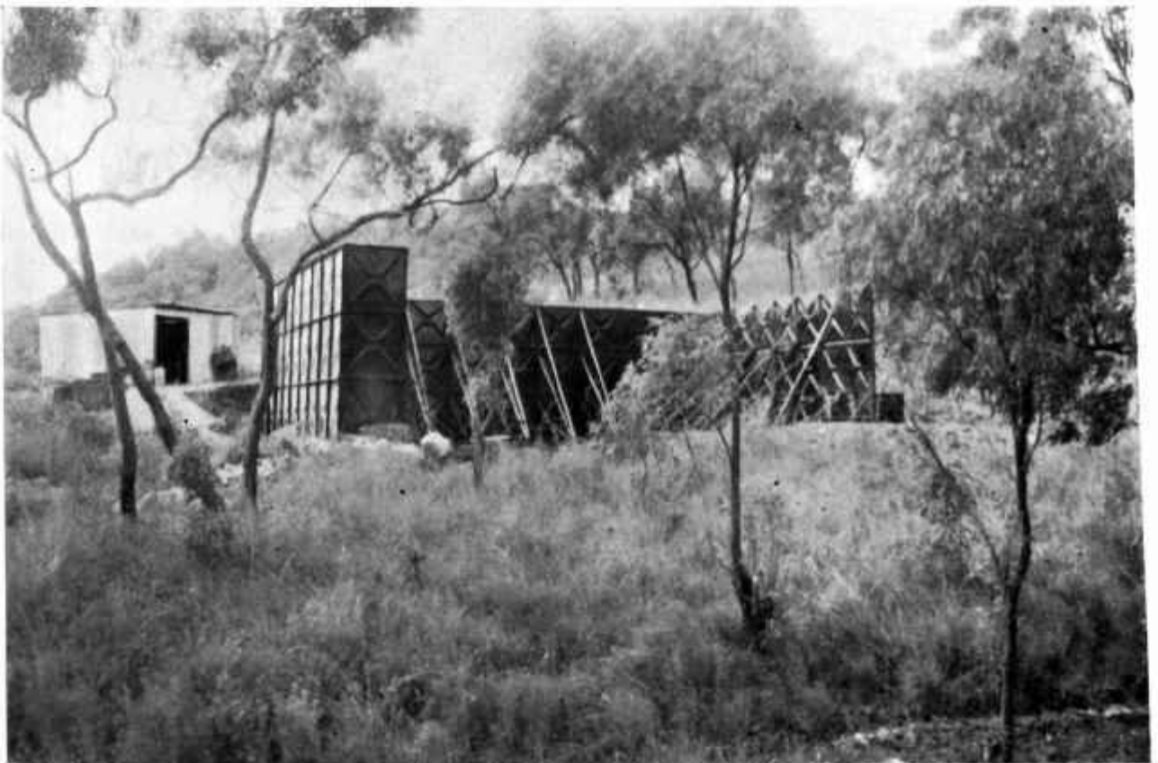
Construction Steel Tanks, Fantome Island Water Supply.
